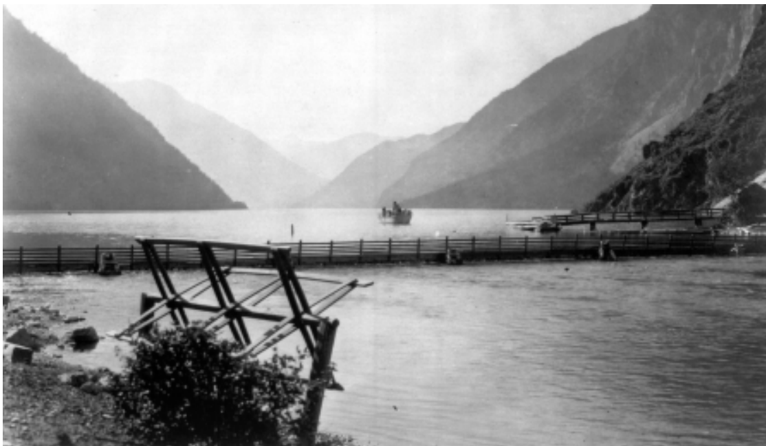
Salmon Weir at Outlet of Seton Lake in 1911 (BC Archives)
